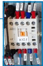
The thermostat is configured at  $-15^{\circ}\text{C}$ . If temperature is lower than this value, contactor will open.
