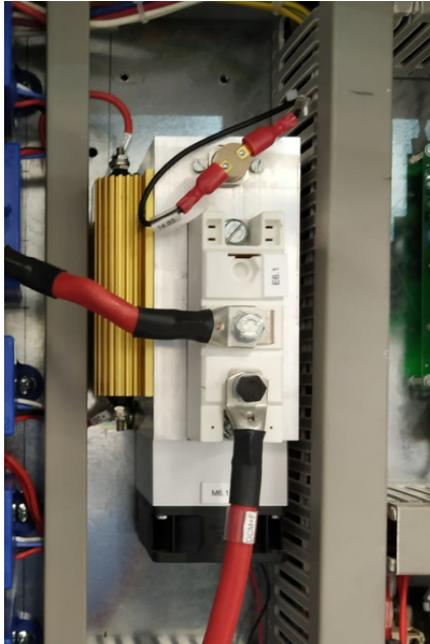
In order to keep a safe temperature in this zone, it is installed a radiator and a fan.
